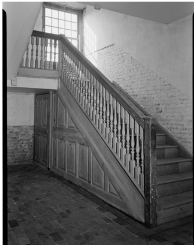
1959 HABS Photo. Of Hall Stairway. A number of the restoration needs are shown. Missing wainscoting requires replacement and paint requires removal on stairway banister. The brick hallway floor has been laid.
